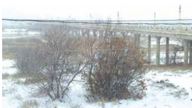
Balcony view of the Fourth Street Bridge and ravine.
